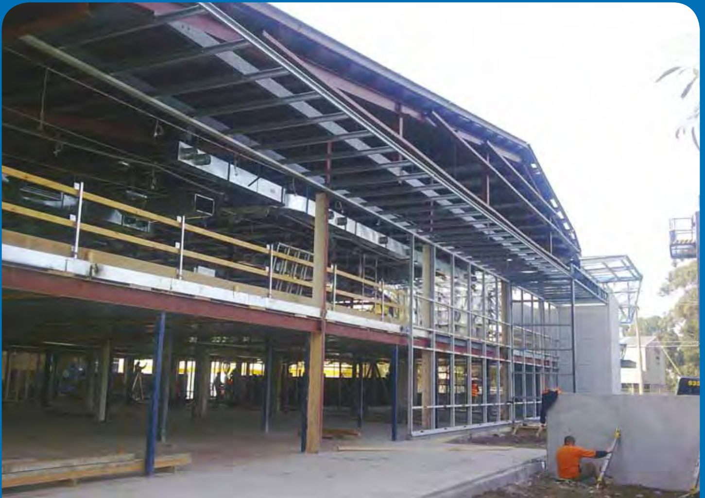
Melbourne Site under construction
