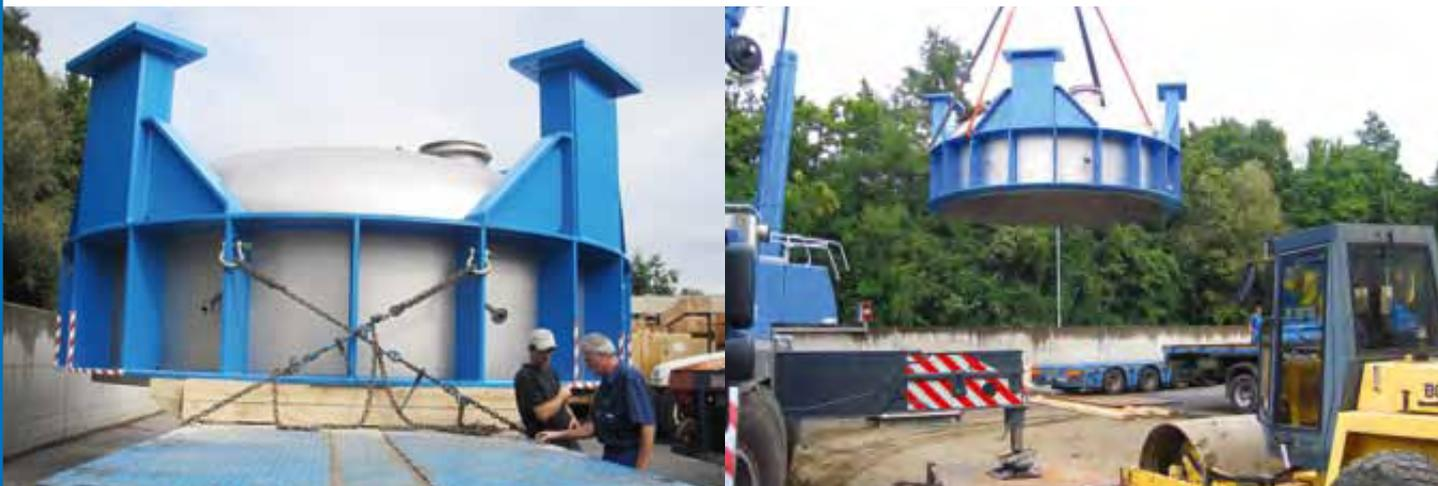
*Loading of the timber processing units in Germany which weigh 35 tonne*
