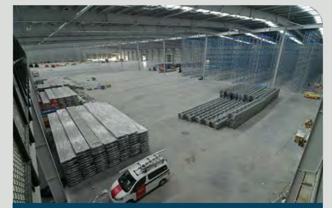
Racking installation underway...55,000 pallet spaces
