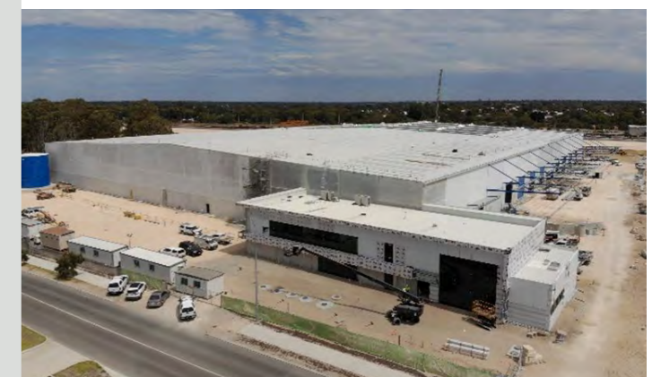
Roe Highway, Perth WA
